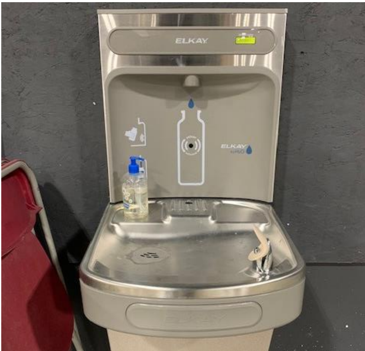
Image of a water fountain with a touchless bottle refill tap. Photo provided by Ontario Green Screen.
